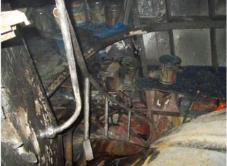
**Figure 10:** The bended bulkhead and the paint buckets found inside the Paint Store.
