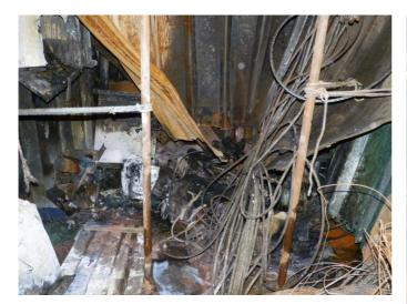
**Figure 6:** Capture of the cracked bulkhead of the Paint Room after the extinguishing of the fire. It is evident that the intermediate (between Paint Room and Boatswain's Store) bulkhead has been heavily buckled by the explosion, blocking the access to the lower space, while the door has been deformed by the explosion gases.
