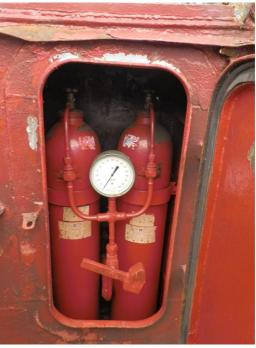
Figure 22: The fixed  $CO_2$  fire extinguishing system located outside of the Paint Room door.
