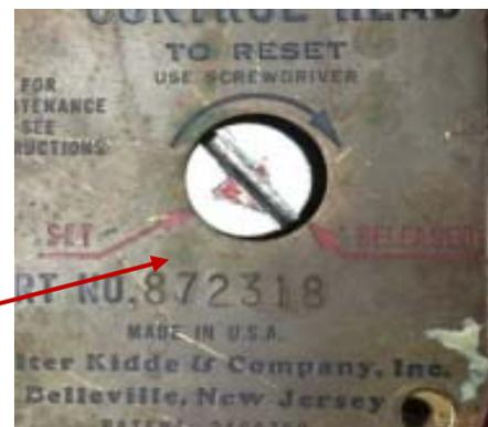
*The slot and arrow indicator on the reset component above aligns with the status of the CO<sub>2</sub> bottle.*
